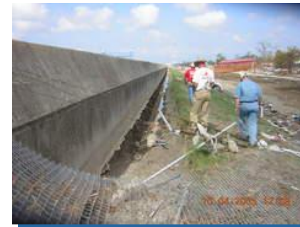
Engineers examine the scoured trench behind the concrete floodwall next to the catastrophic levee breach at the west end of the Lower Ninth Ward of New Orleans. Credit: Rune Storesund
