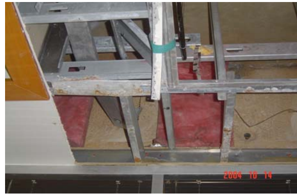
Figure 9: Mold Remediation Project
