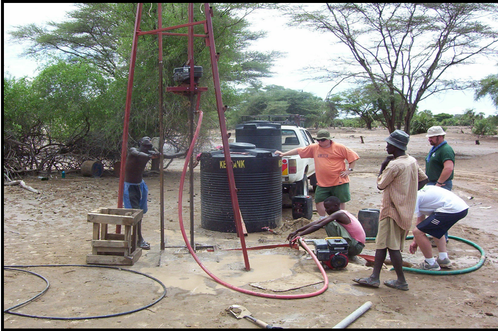
Figure 3: Drop Hammer
