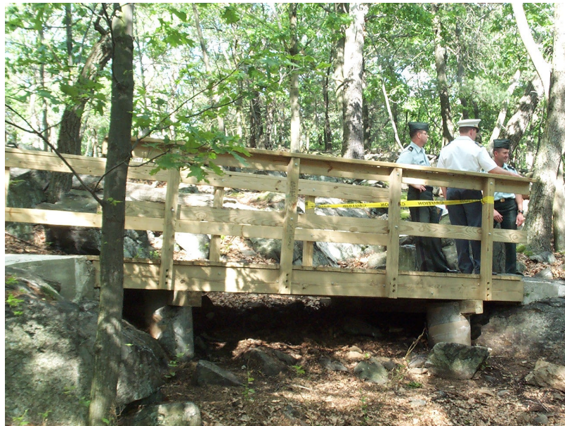
Figure 4: Finished 16 foot span
