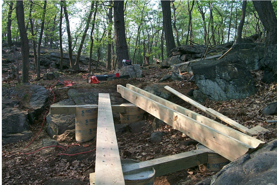
Figure 3: 6”x6” lumber cradled placed in two concrete Sonoform ® tubes
