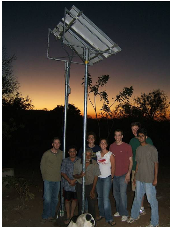
Figure 5: Solar panels and project team
