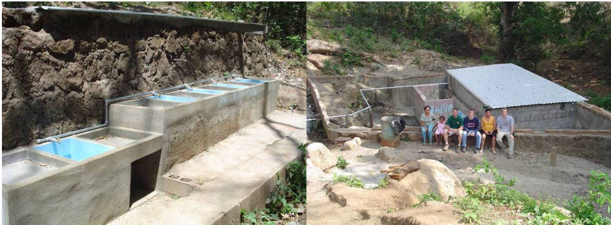
Figure 3: Completed washing stations and water storage tank
