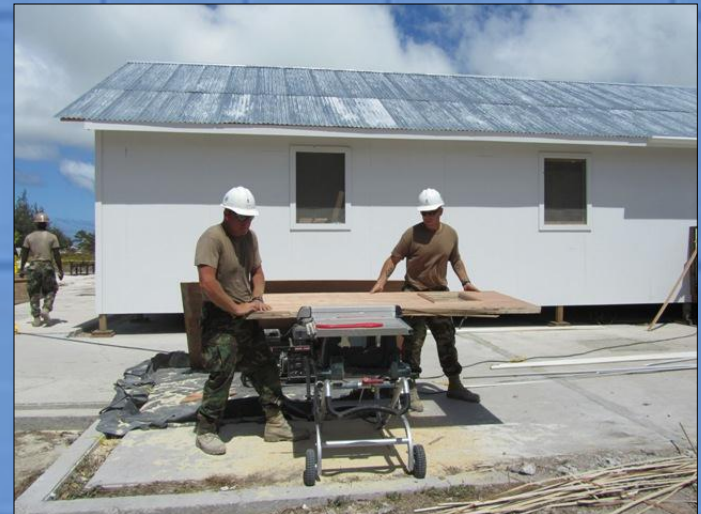
CCAD Kiribati constructing the Maternity Clinic
