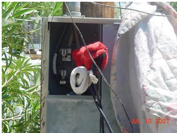
Figure 5. Examples of bypassing a metering through the use of automobile jumper cables (a) and screwdrivers (b), from [7].
