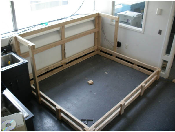
Figure 12 Basin under construction
