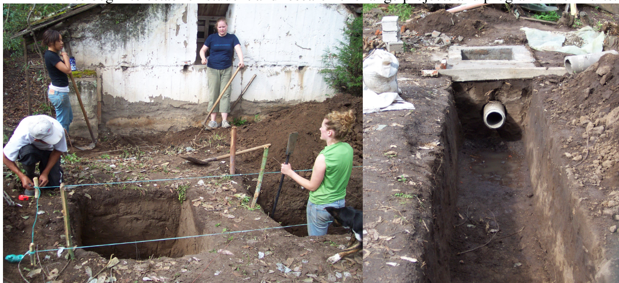
Figure 3 Construction of Bio-Gas Trench Unit in Ecuador
