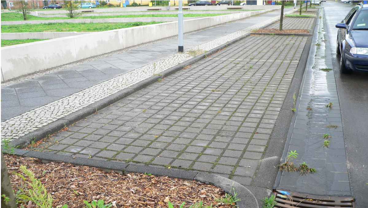
Picture 3: Grid-Brick pattern allowing water to drain into ground
