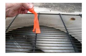
Figure 10. Tape held at center of fan showing vacuum.
