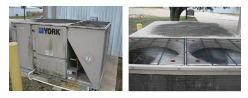
Figure 3. R-410A XP series 6-1/2 ton 60Hz AC Condenser Unit
