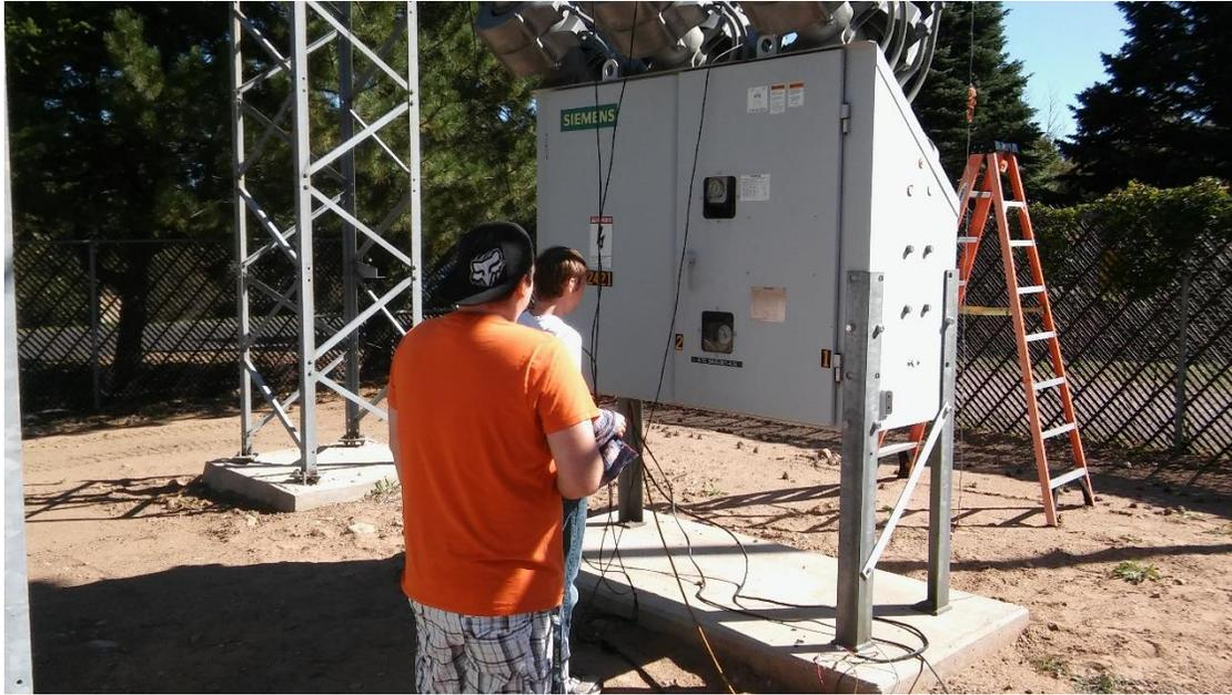
*Figure 5. Students Testing the 72.5 kV Puffer SF6 Circuit Breaker*
