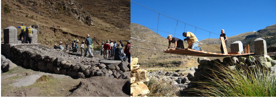
Construction of right abutment ramp
