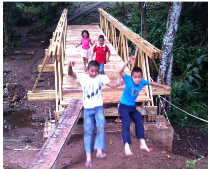
Fig. 9. Local children enjoying the nearly completed bridge.
