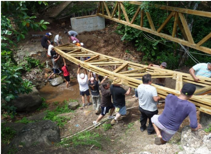
Fig. 7. Moving the completed trusses into place at the site
