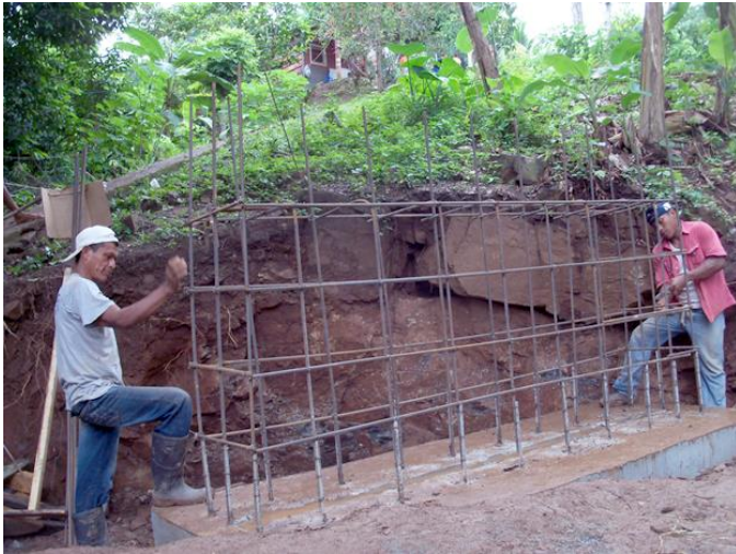
Fig. 6. Foundation and abutment construction – cast-in-place concrete with reinforcement
