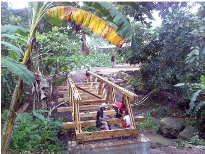
Fig. 8. Floor system construction
