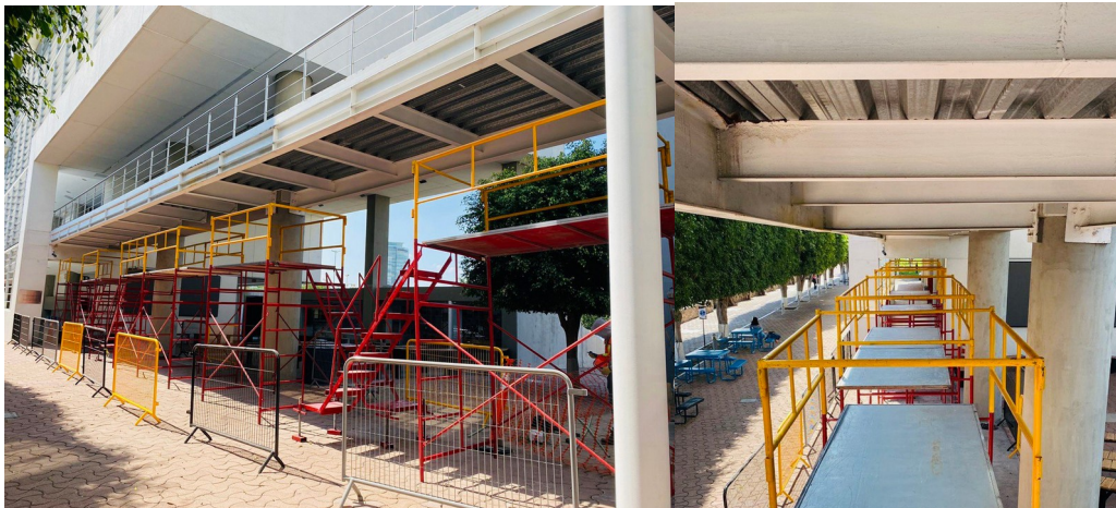
Fig. 5 Steel bridge in Campus BBBB.
