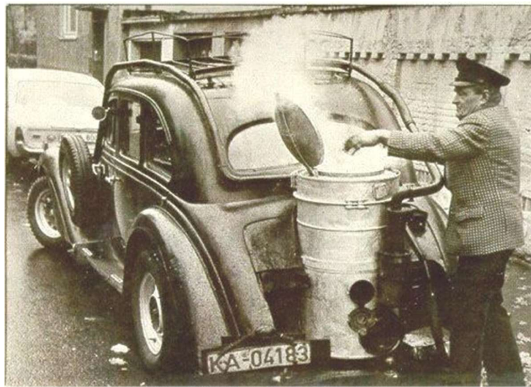
Figure 1. Photo of a WWII era German vehicle with wood gasifier fueling unit.
