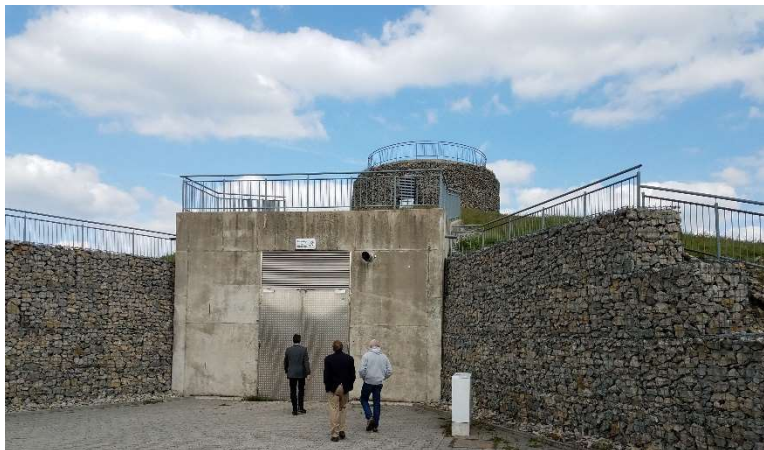
Figure 9. Surface entrance to the Crailsheim underground seasonal energy storage system.
