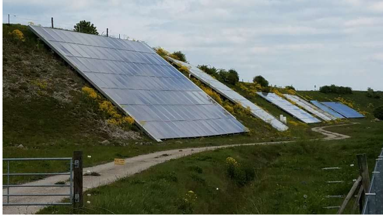
Figure 8: In the German town of Crailsheim, 7,300 m 2 of solar thermal flat plate collectors provide 50 % of the heat for 260 homes. Heat energy is captured and stored seasonally in a 37,500 m 3 underground thermal borehole system.
