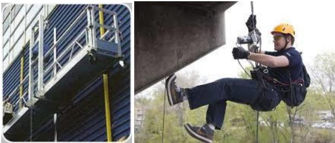
Fig. 1. Suspended platform inspection (Left) and grappling inspection (Right)
