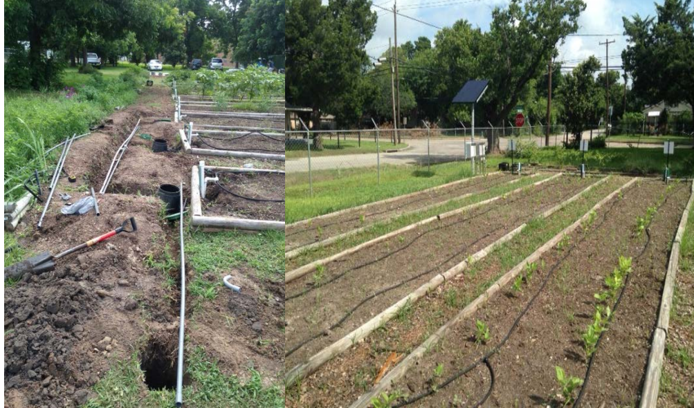
Figure 3: Installation of Community Garden Irrigation System and Solar Panels
