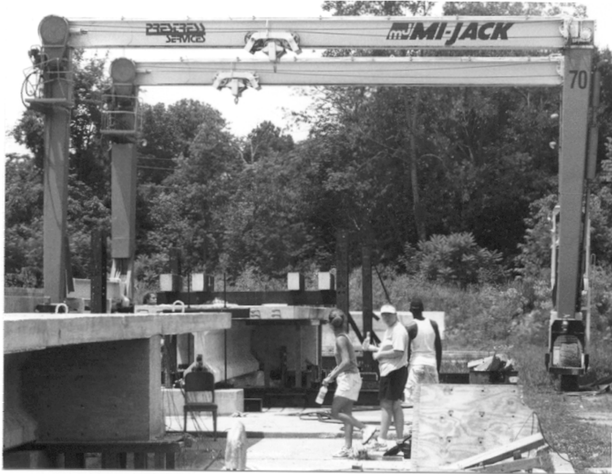
Figure 1. Prestressed Concrete Group Preparing for Testing
