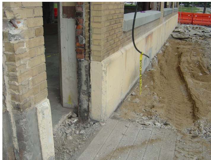
Figure 3: Site Photo of Wall/Floor Intersection
