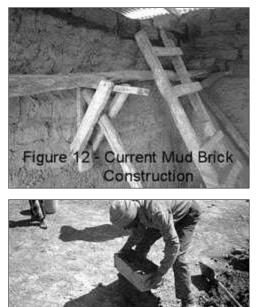
Figure 13 - Making Mud Bricks
