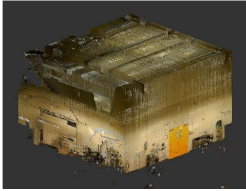
(a) Exterior View
