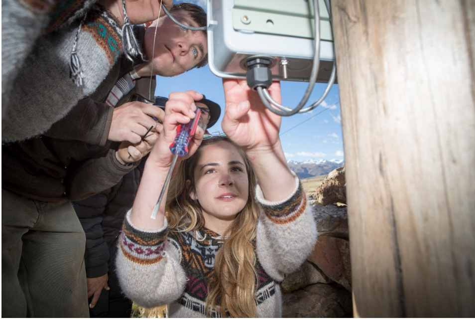
Students installing the Appalachian Street Lamp in a remote village in Peru
