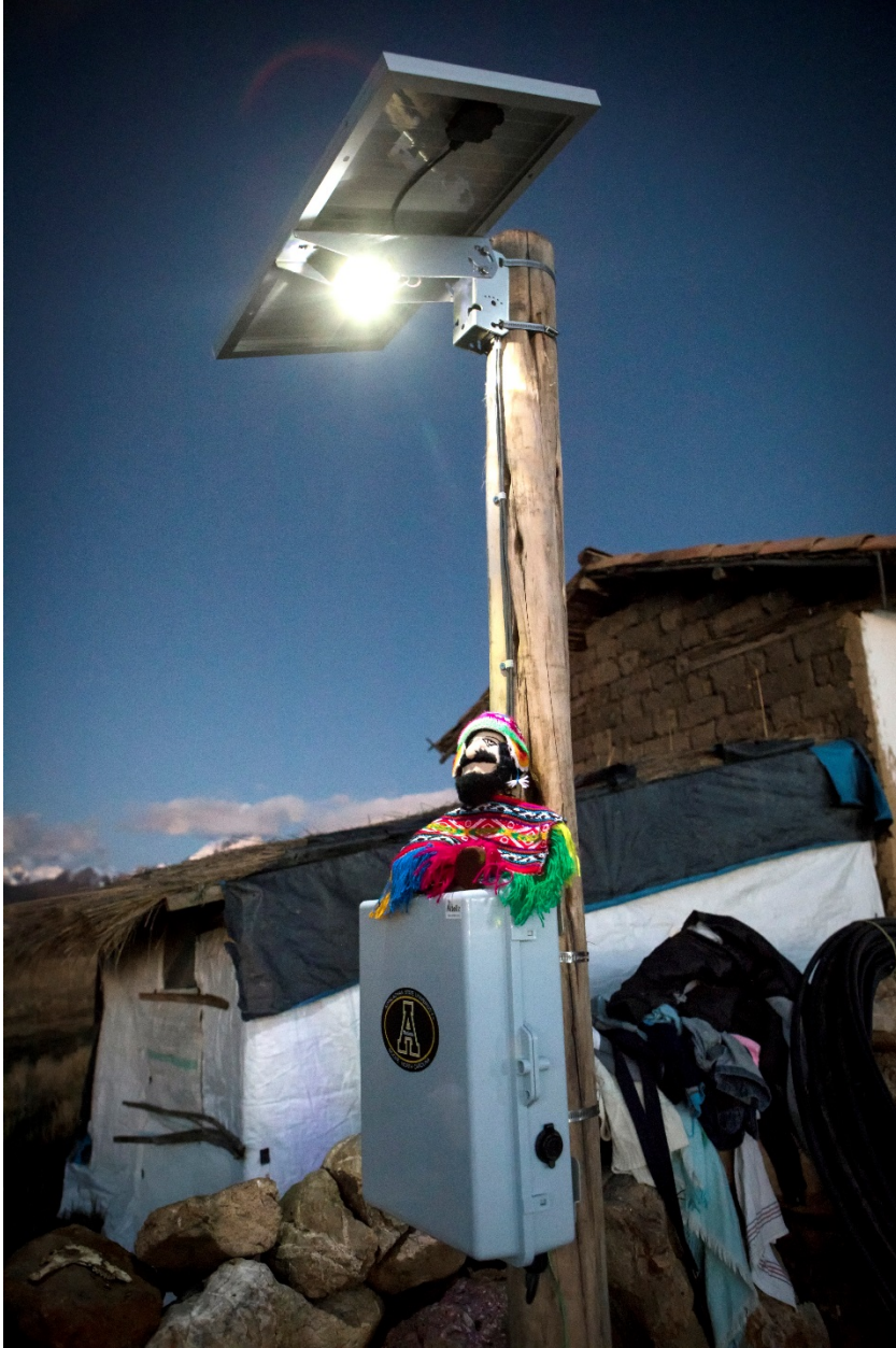
Appalachian Street Lamp operating in a remote village in Peru (with Yosef)
