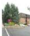
Fig. 1 This is a picture of the home that we are converting to 50% natural gas and 50% solar power. The home is located in Belleville. It is 1200 ft 2 and three people live here.
