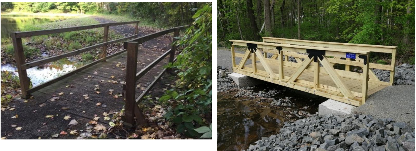
Figure 5: The Previously Existing Bridge and the New Bridge
