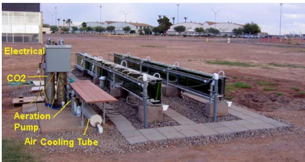
Figure 4: The AzTE reactor from the northwest, and after landscaping. The wet ground resulted from a spill, not from leakage.
