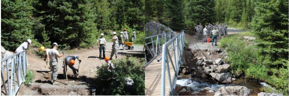
Figure 10. “By-hand” excavation of the north side of the bridge
