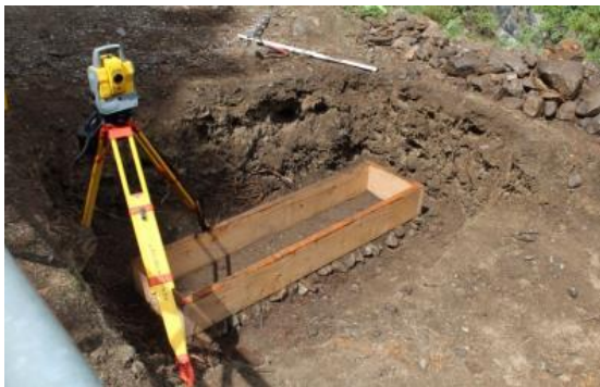
Figure 12. One of the bridge abutments with a concrete form in place
