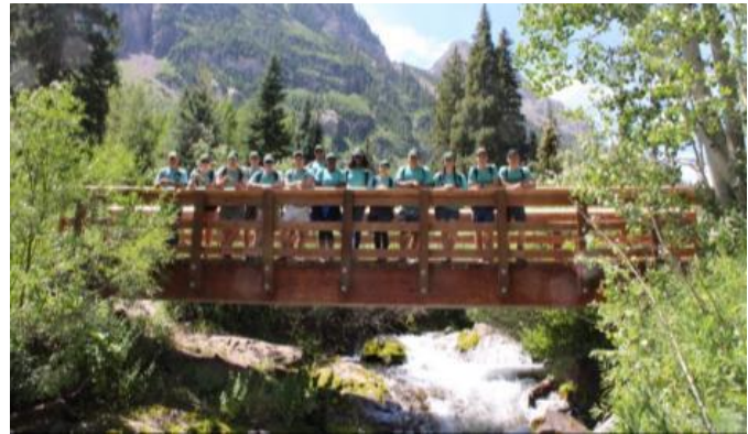
Figure 7. Maroon Bells glulam beam, constructed by USAFA Class of 2017
