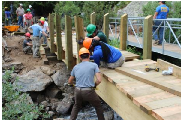
Figure 16. Decking and rail posts are being installed
