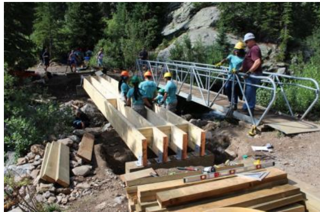
Figure 15. Stringers in place with diaphragms being installed
