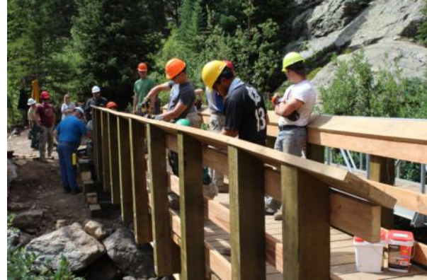
Figure 18. Railings and rail caps installed
