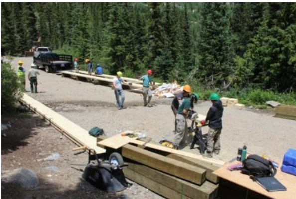
Figure 13. Prefab location, just down the hill of the bridge site
