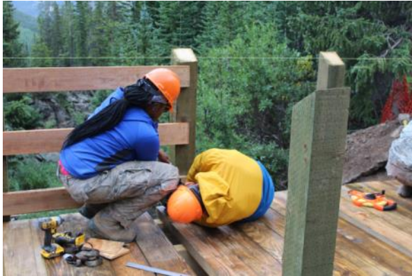
Figure 17. Railing measuring and installation
