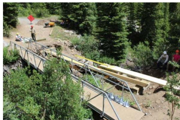
Figure 14. Rigging setup used to lift the stringers across the stream
