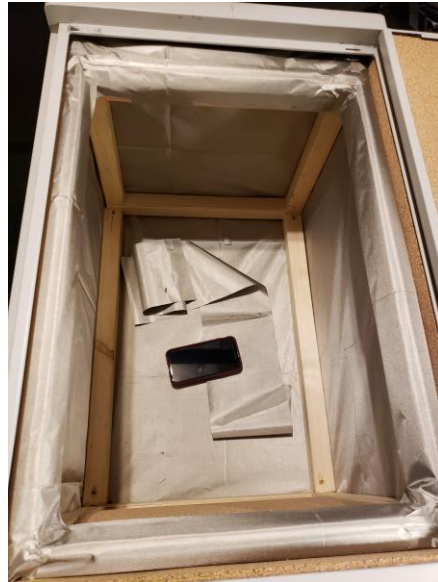
Figure 6: Supports Insulated in the Cabinet
