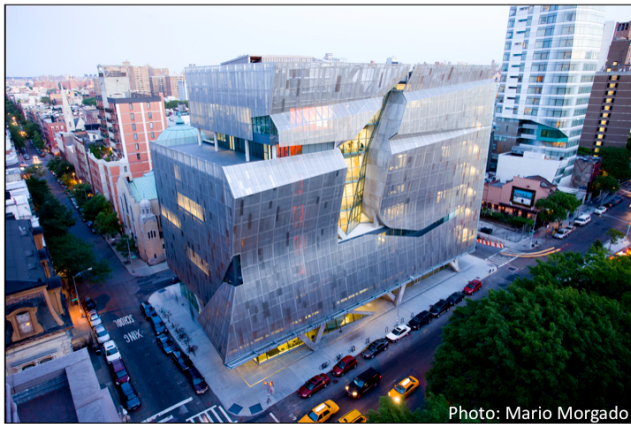
Fig. 1. 41 Cooper Square. A new LEED Platinum certified academic building is used as a context to explore control system concepts.
