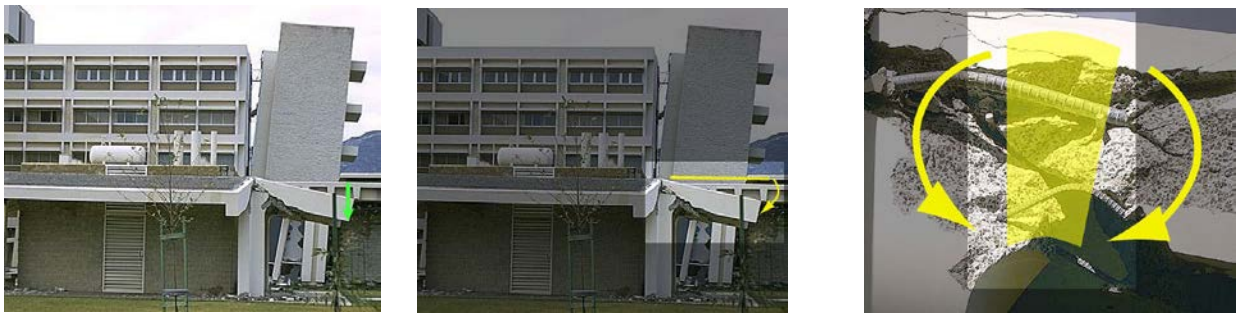
Figure 3-2 The bending failure of the canopy due to seismic tremor can better be understood by changing viewpoints.
