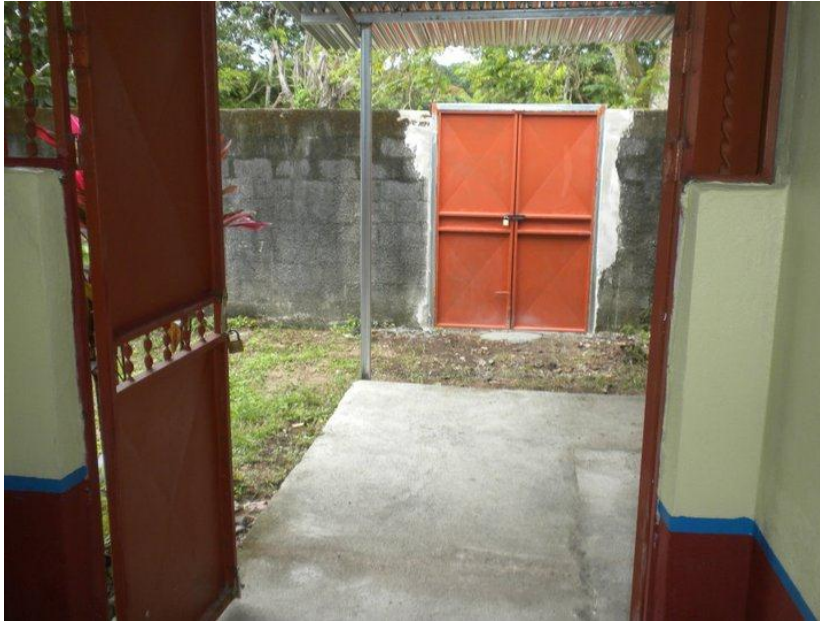
Figure 3: Emergency exit for health clinic in Costa Rica
