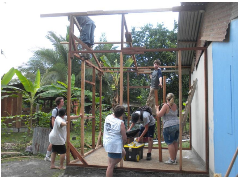
Figure 2: Room addition on home in Costa Rica
