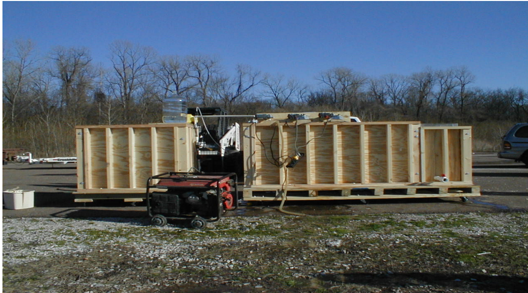
Figure 7 Picture of Completed System at the Mississippi River
