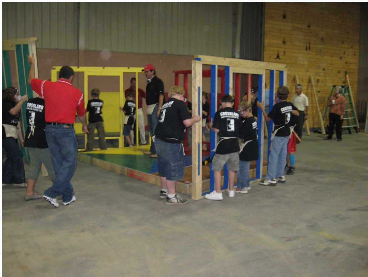
Installing wall framing
