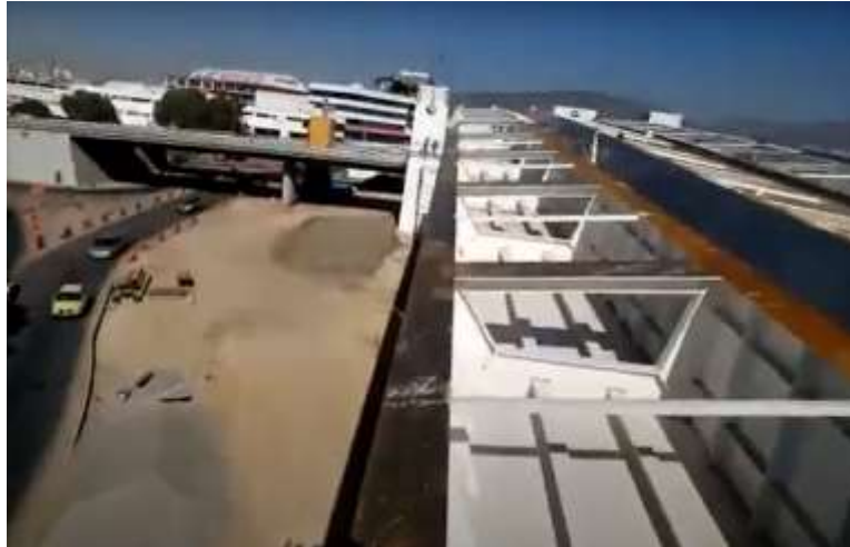
Figure 9. Zoom visit to a cable stayed bridge
