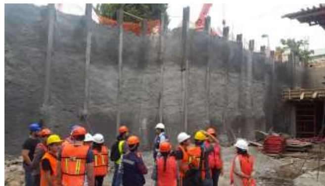
Figure 8. Site visit to a retaining wall construction using “Berlin” system.
