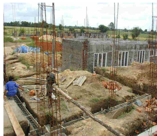
Figure 7: Plinth Beam overview
