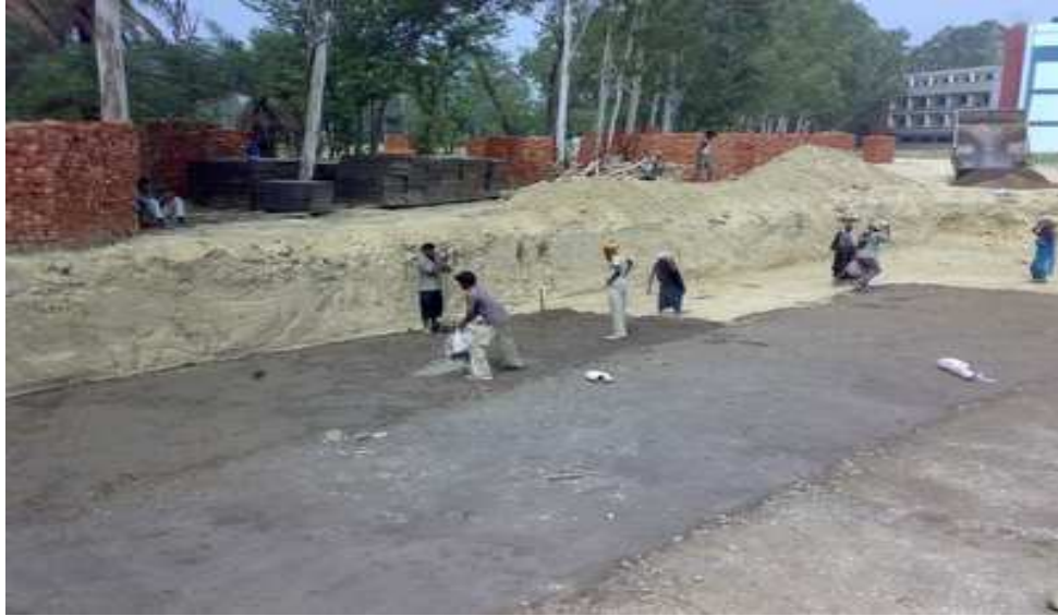
Figure 3 Laying of P.C.C
