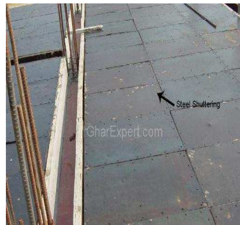
Figure 9: Shuttering plates set for slab
