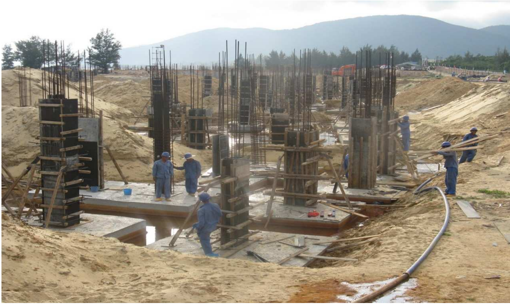
Figure 5 Erection of Columns
