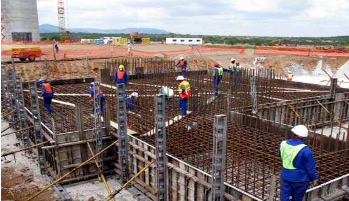
Figure 4 Laying of Foundation
