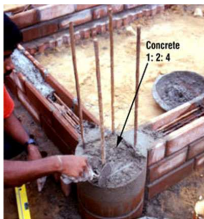
Figure 6: Concreting of plinth beam
