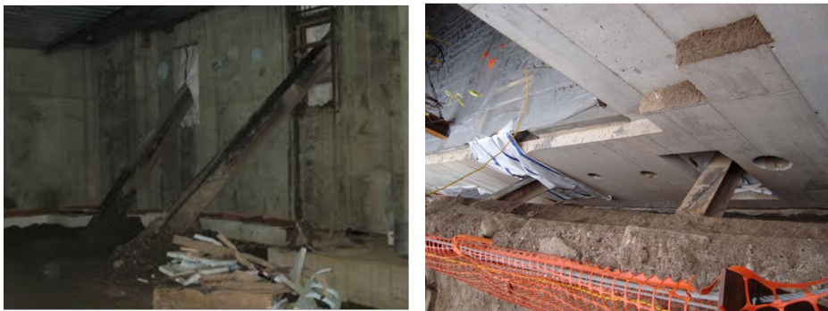
Figure 26. Raker system (Photos used by permission)
