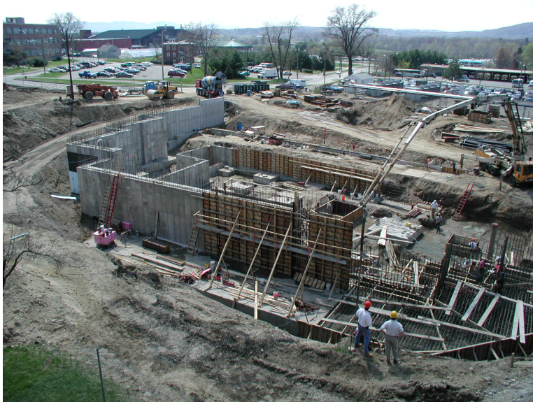
Figure 31. Site work and concrete foundations (Photo used by permission)
