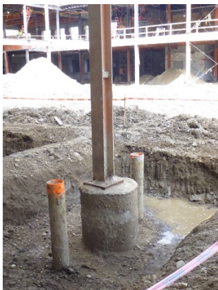
Figure 30. Existing foundation with new micropiles (left) and completed footing (right)
