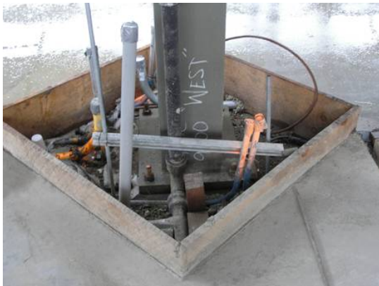
Figure 10 Boxout for baseplate (Photo used by permission)
