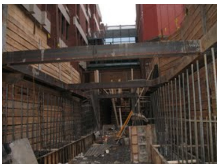
Figure 27. Trench supports (Photo used by permission)
