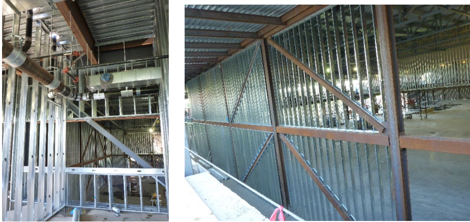
Figure 19. Non-structural wall framing (Photos used by permission)
