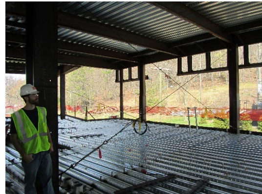
Figure 8. Temporary bracing (Photo used by permission)
