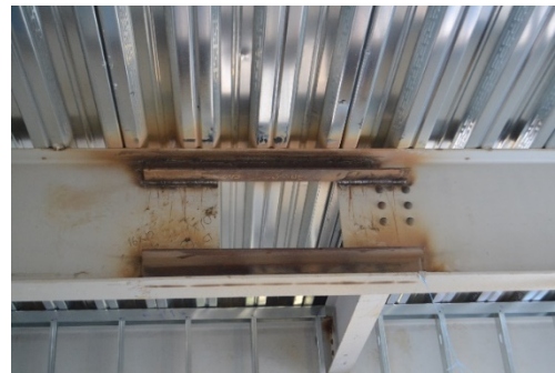
Figure 18. Field fix for HVAC (Photo used by permission)
