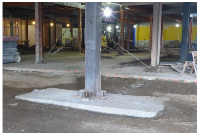
Figure 30. Existing foundation with new micropiles (left) and completed footing (right)
