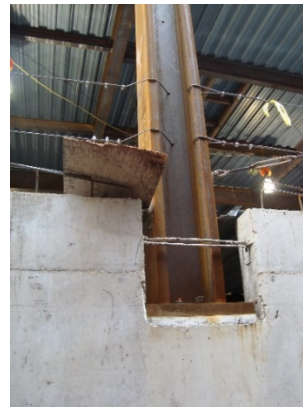
Figure 11. Perimeter column baseplate (Photo used by permission)
