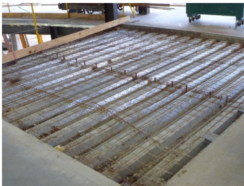
Figure 7. Composite slab details (Photo used by permission)
