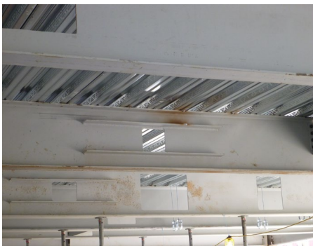
Figure 17. Coordinated HVAC design (Photo used by permission)
