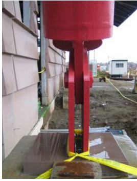
Figure 14. Pinned connection connections (Photo used by permission)
