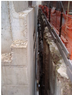
Figure 25. Secant piles (right side) (Photo used by permission)
