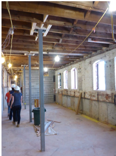
Figure 28. New steel LFRS (Photo used by permission)
