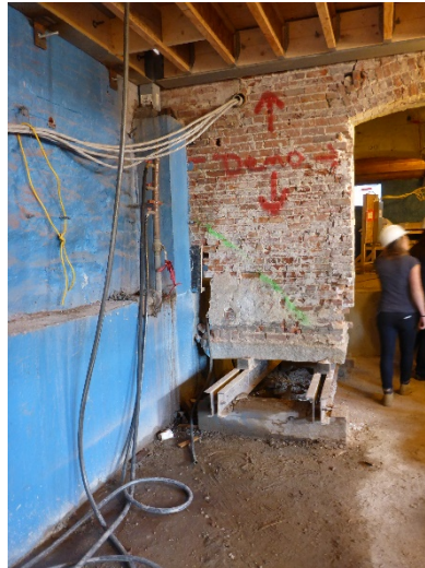
Figure 29. Underpinning of existing wall (Photo used by permission)
