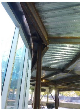
Figure 12. Curved façade framing (Photo used by permission)
