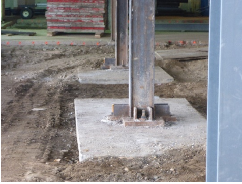
Figure 9. Spread Footings (Photo used by permission)
