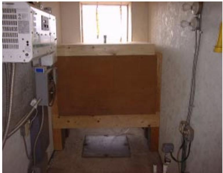
Figure 4. New Battery Box in the Pump House. Inverter-Controller is at Upper Left of Picture
