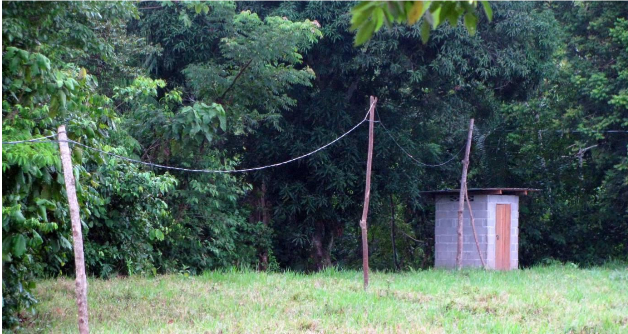
Figure 4: Madreado tree branches used as electricity poles.
