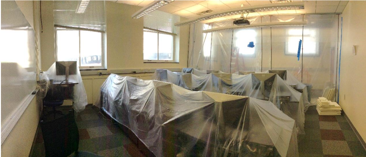
Figure 1: The computer classroom right after the wall was removed.
