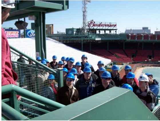
Figure 2 – students tour the Fenway Park Renovation with Shawmut Construction of Boston, Massachusetts in 2008
