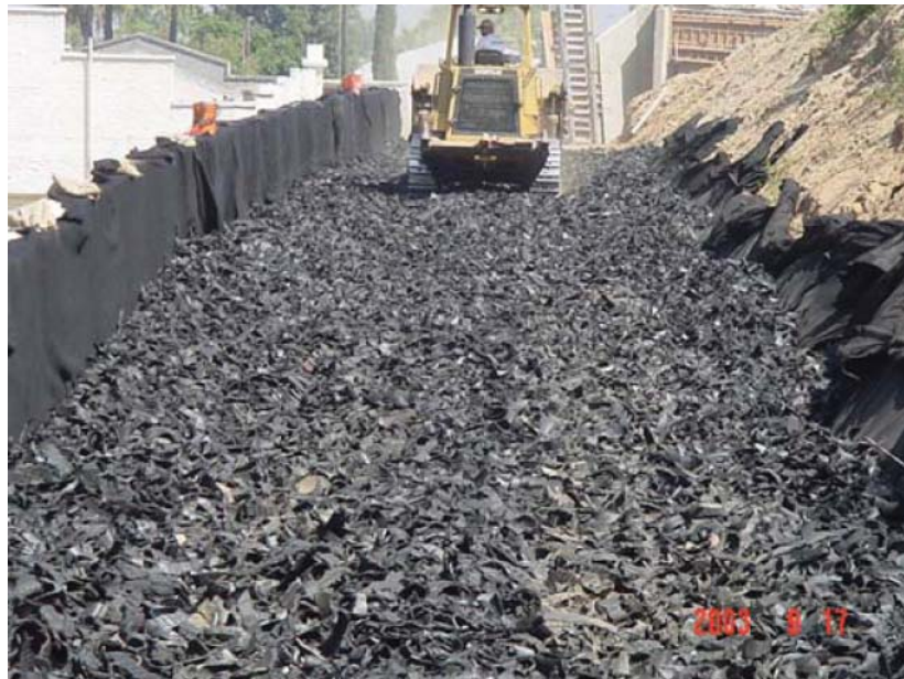
FIGURE 2. TDA as Backfill for Retaining Wall 119 in Riverside, CA (15)
