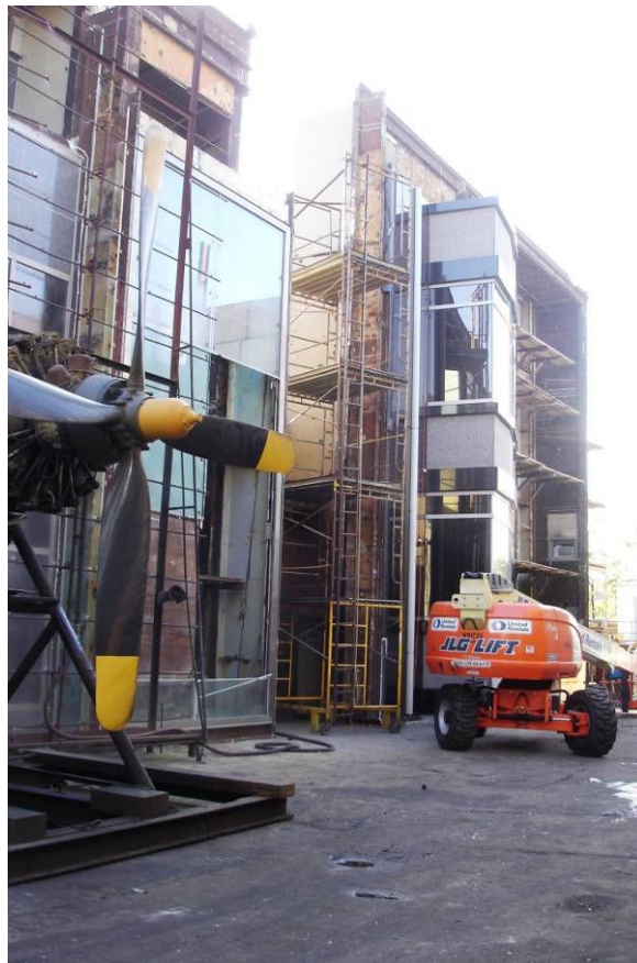
Figure 4: Curtain wall mock-up
