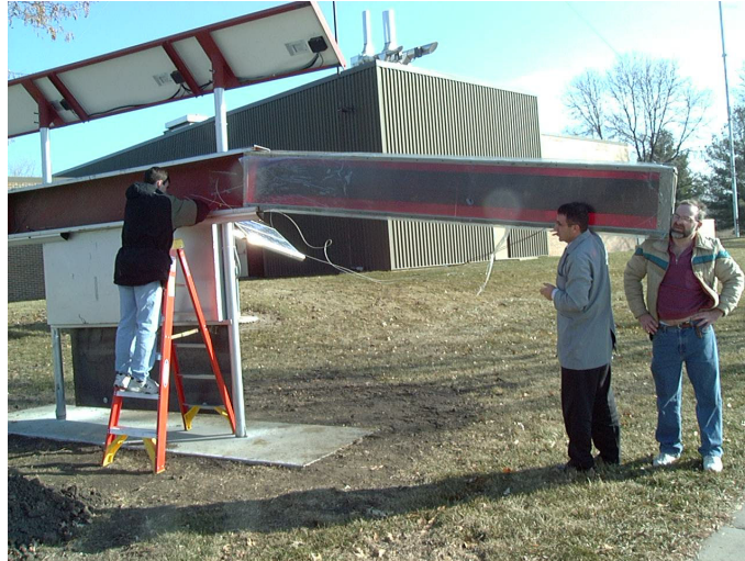
Figure 4. Installation of outdoor digital display into the metallic frame
