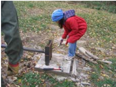
Figure 5. Pounding in base pivot pin
