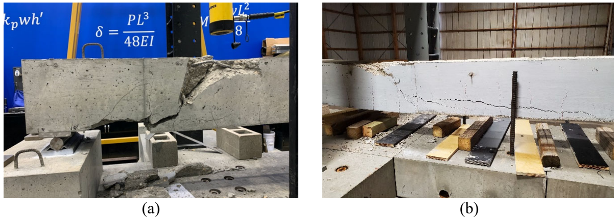
Figure 10—(a) Shear Analysis and Design Specimen at SLU with intentional design flaws and (b) the final resulting failure location (a delamination failure) of the shear specimen at RHIT
