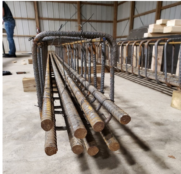
Figure 6—Rebar ties used to connect stirrups with longitudinal reinforcement.
