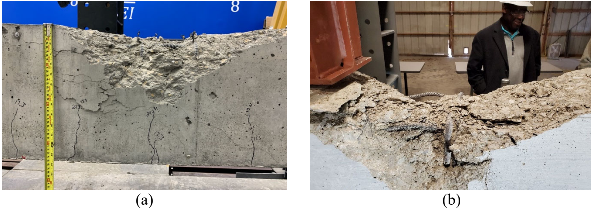
Figure 9—(a) Depth of compression zone of SLU beam and (b) the resulting failure location of RHIT beam.
