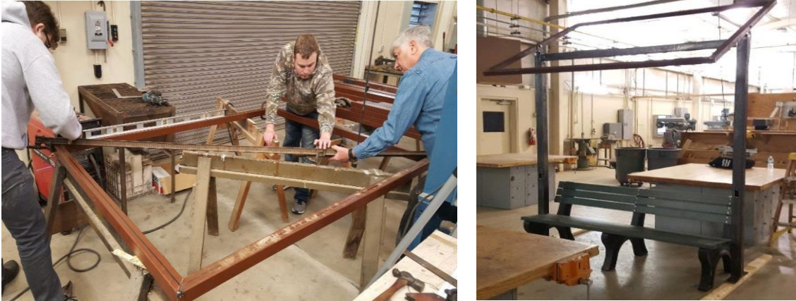
Figure 7. (a) Reinforcing of the metal frame of the charging stations, (b) bench charging station frame was completed
