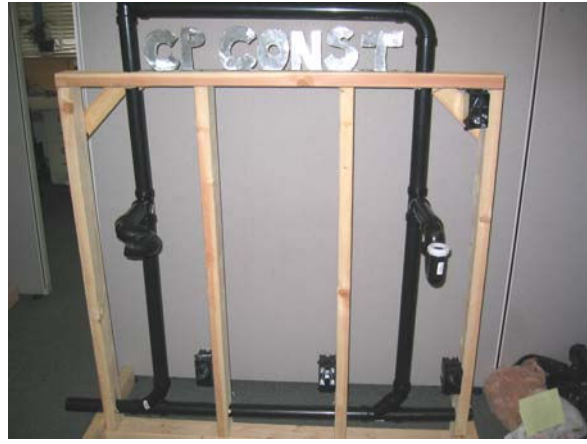
Photo 2 and 3 –Workstation with Drainage System Installed and Electrical Rough-in Started
