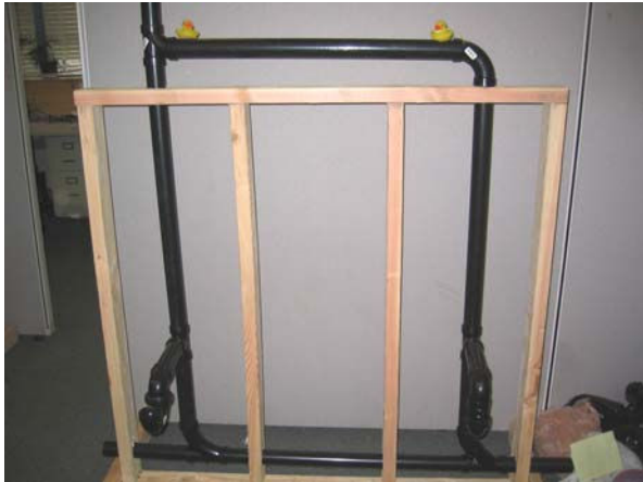
Photo 2 and 3 –Workstation with Drainage System Installed and Electrical Rough-in Started
