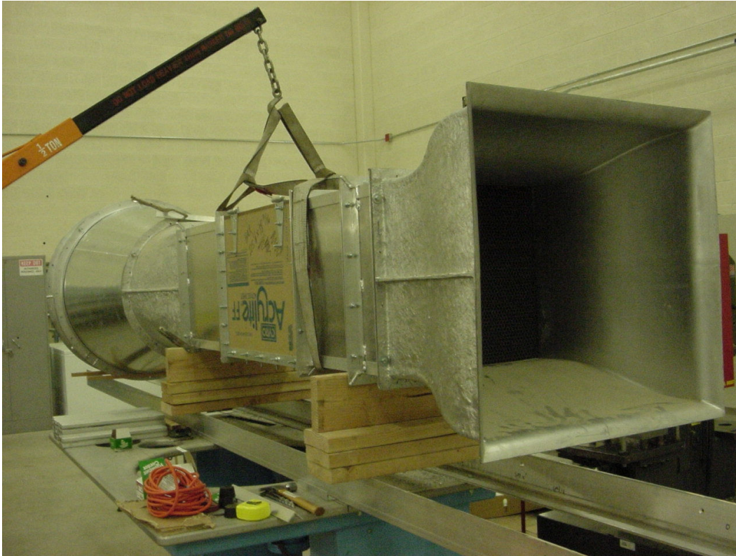
Figure 2 – Wind Tunnel under Construction
