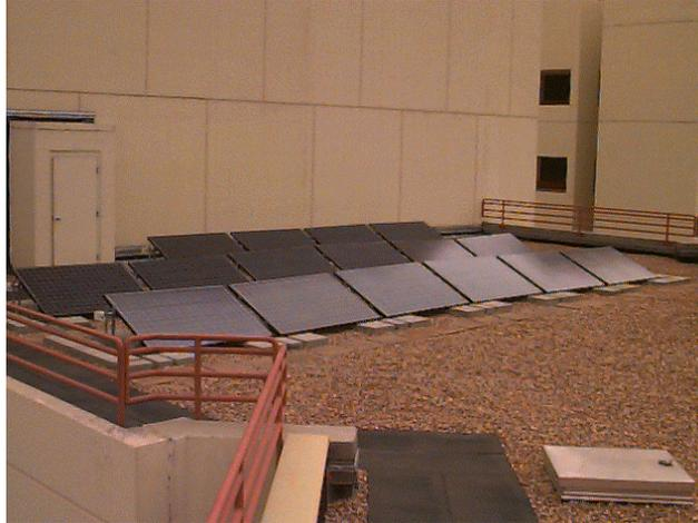
**Fig. 2. The 5 kW Rack-mounted PV array**
