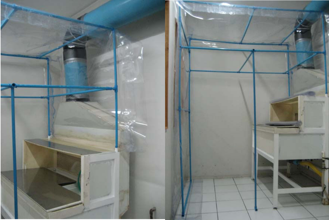
Fig. 1. Two views of the refurbished wet-etch station with exhaust pipe installed. The stainless steel work surface and sink are visible in the photo on the left.
