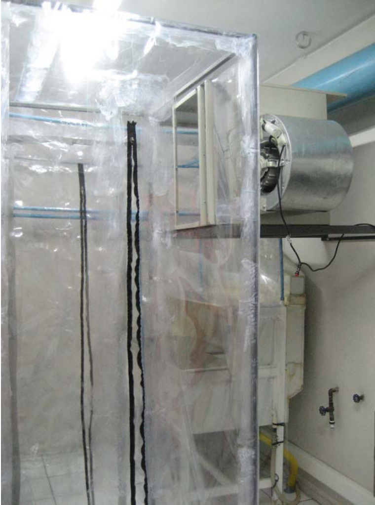
Fig. 3. The anteroom to the cleanroom with zippered entrance.
